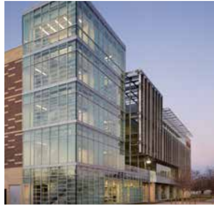
▲ Modern high school. A smart combination of horizontal and cantilevered CS Airfoil® blades protect interiors from heat and glare while adding a distinguishing touch to the building.
