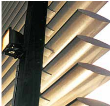
▲ Birdsmouth brackets. Horizontally mounted CS Airfoil® AF270 blades and their mounting structure shown from behind. Birdsmouth brackets have been fixed onto vertical support segments at specified distances and CS Airfoil® blades were then simply slotted into the brackets and fixed with screws or rivets. Birdsmouth brackets allow for speedy onsite installations and have the additional advantage of being virtually invisible when seen from the front.
