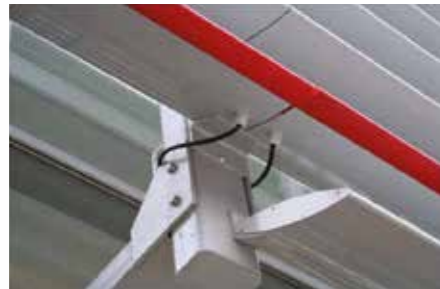
▲ Power supply. CS Airfoil® LUX® illuminated blades are supplied with 12 V low voltage transformers accommodated inside the building.
