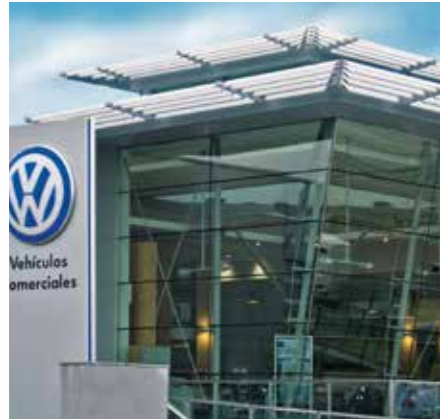
▲ VW show room. CS Airfoil® blades in a cantilevered solar protection system in front of the glass facade of a VW car show room.
